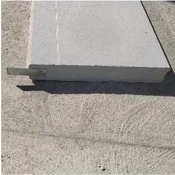
STEP 2 ▶ GX500 application before install wall panel
