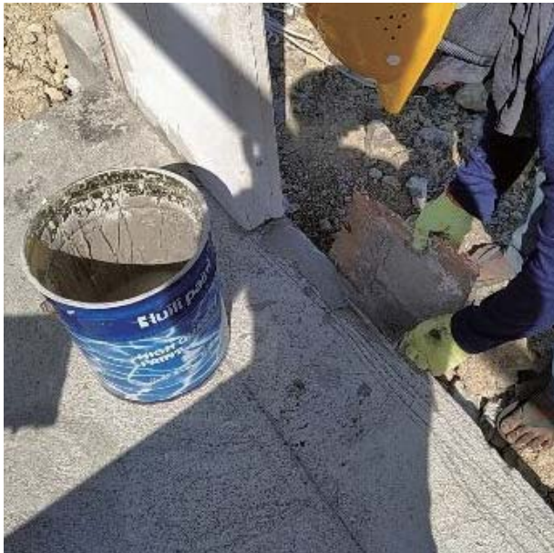
◀ STEP 3 ALC panel installation and push together
