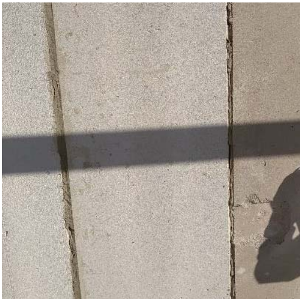
◀ STEP 3 ALC panel installation and push together
