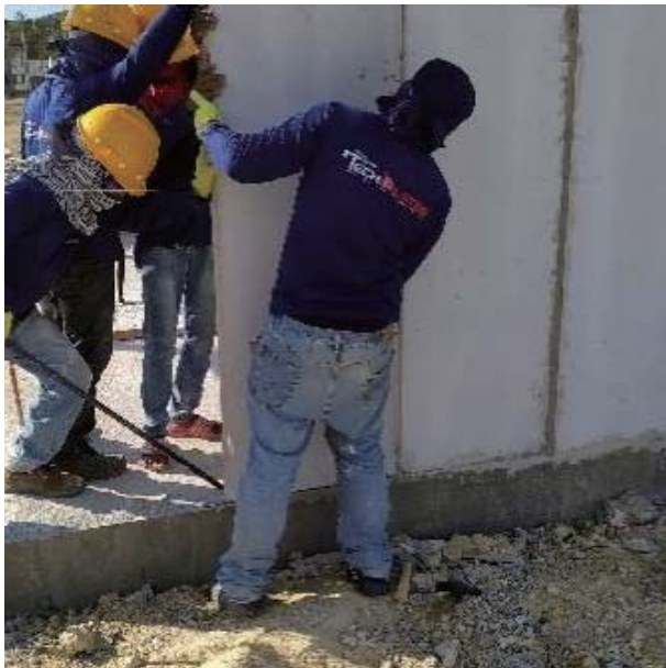
STEP 4 ▶ After fixing of ALC wall panel
