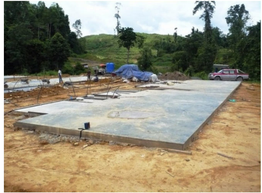
2.) Casting of Raft Foundation
