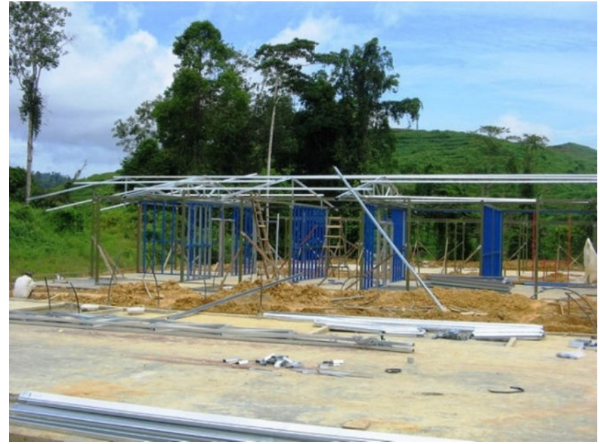
4.) Metal frame installation and Steel trusses
