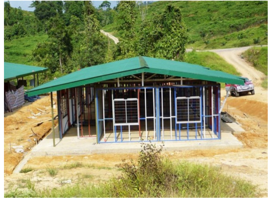
5.) Roofing installation and Wall Framing Closure
