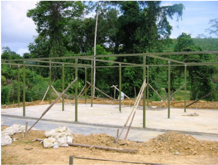
3.) Erection of Steel Columns & Beams
