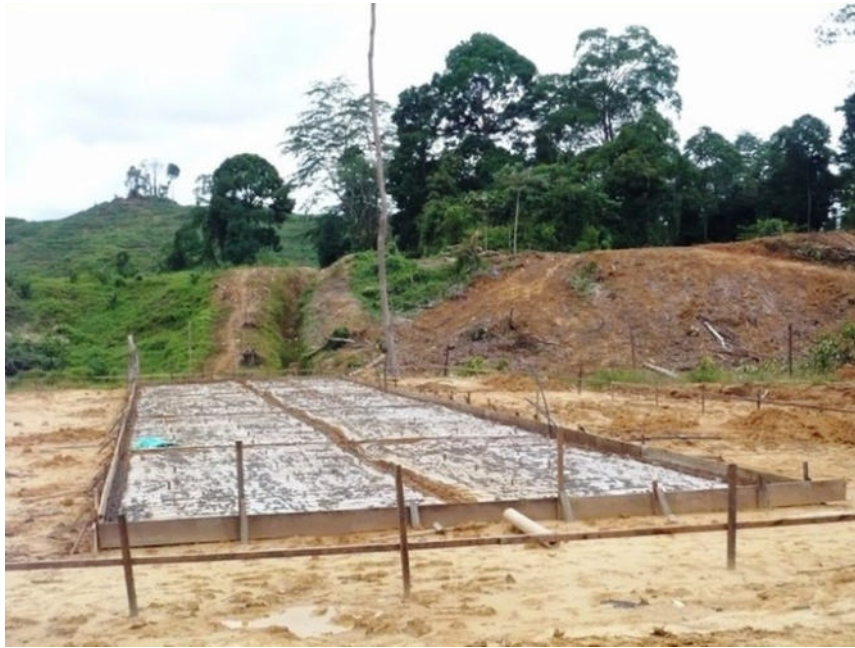
1.) Formworks at Raft Foundation
