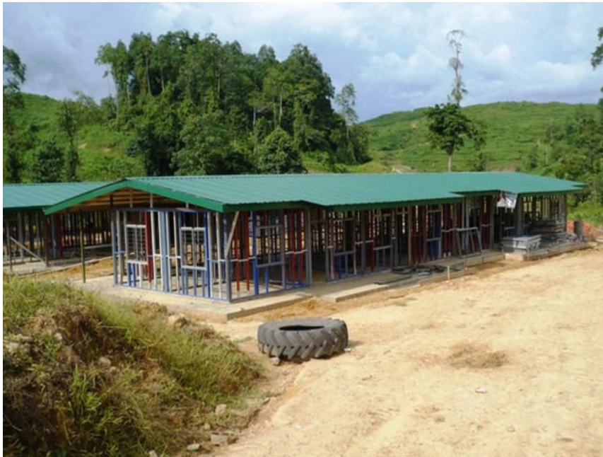
5.) Roofing installation and Wall Framing Closure
